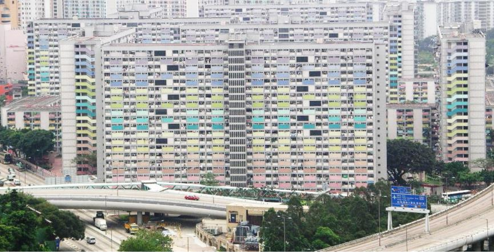
Slab Block (1960s) Choi Hung Estate 16-storey Living room + bath room + kitchen
