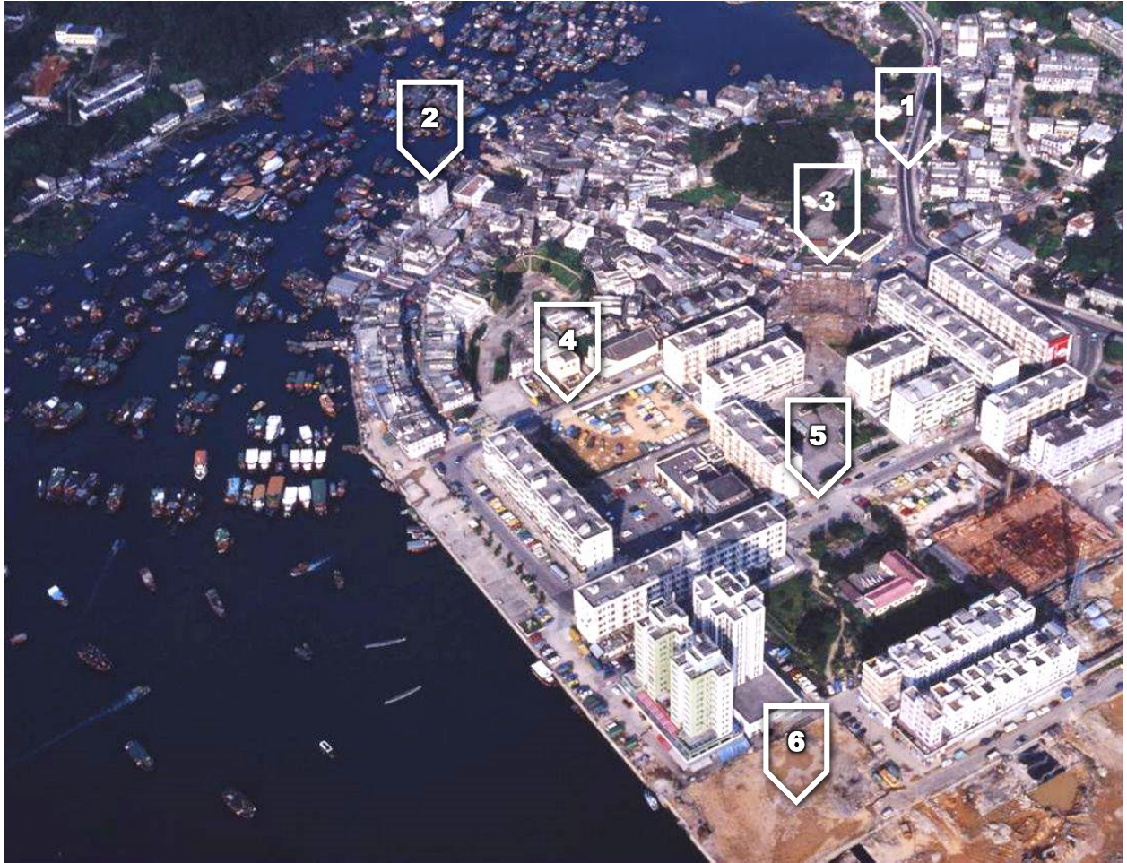
Figure C4: Sai Kung Town, 1983. 1: Hiram's Highway; 2: Kat Cheung Building; 3: Tin Hau Temple; 4: Yi Chun Street; 5: Man Nin Street; 6: Light bus terminal nowadays. New residential buildings on the right foreground were built in 1975 to cater for resettlement due to the construction of High Island Reservoir.
